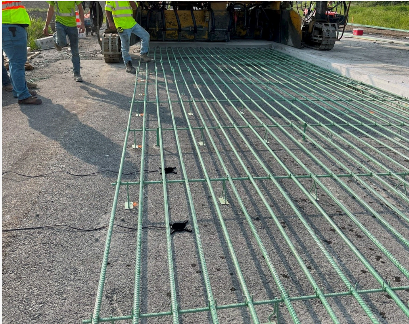
Drop on Roadbed
