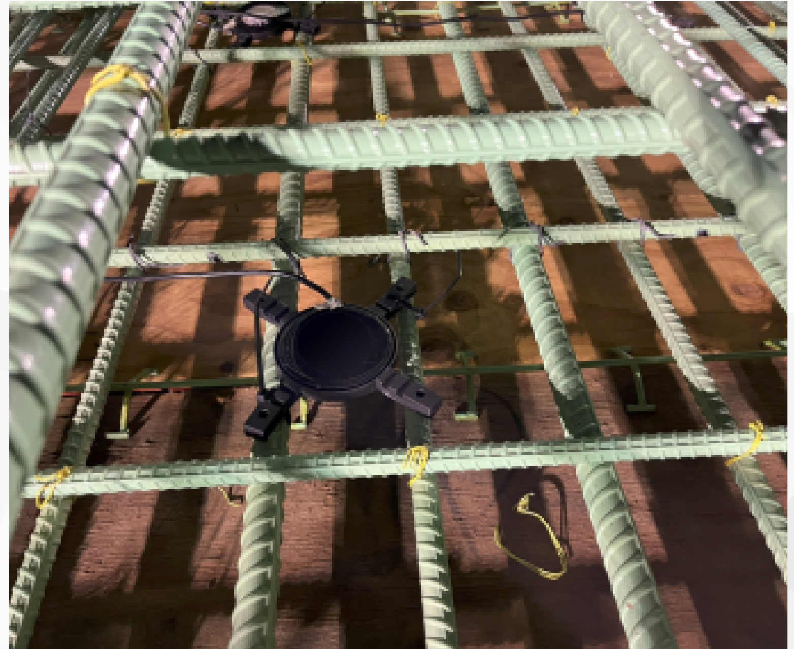
Strap to Rebar
