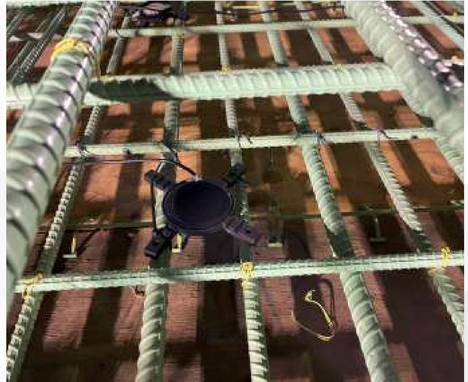
Strap to Rebar
